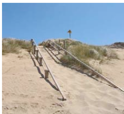
Photo 3-1: Sand build up on beach access steps
