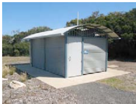
Photo 4-11: Toilet facilities at the Recreation Reserve
