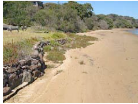
Photo 4-7: Stone sea wall along the creek
