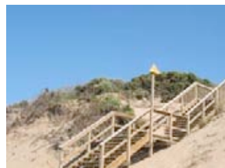
Photo 4-15: Typical beach/dune access steps
