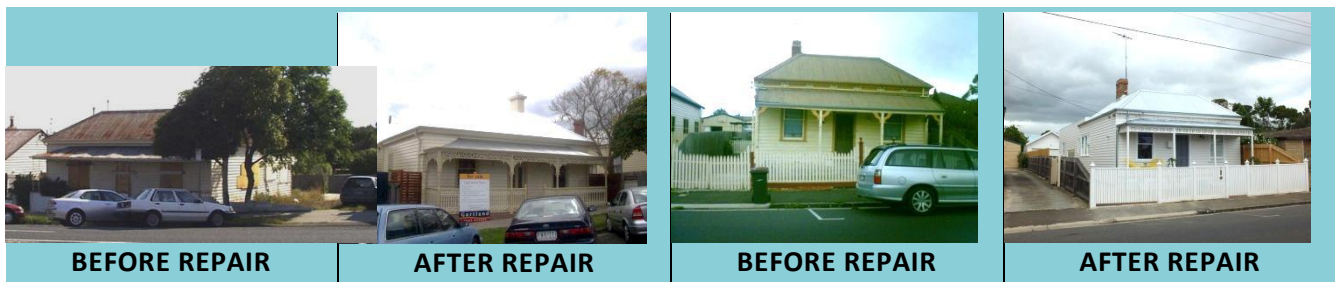
Significant dwellings proposed for demolition and later repaired
