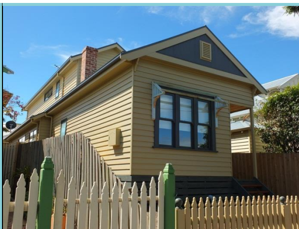
COMPLETED WORKS, INCLUDING SUBSTANTIAL REPAIRS, REAR ADDITIONS AND CHIMNEY RECONSTRUCTION.
