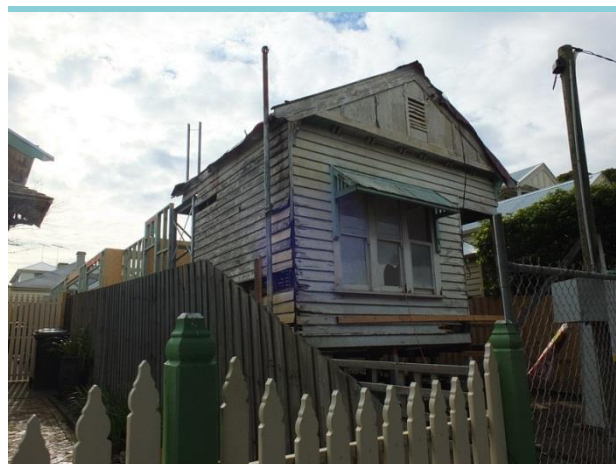
DWELLING TEMPORARILY PROPPED DURING DEMOLITION & CONSTRUCTION.
